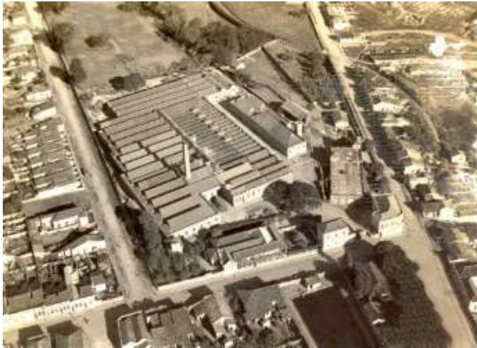
1954 Fábrica Santa Maria Rua Santa Maria
